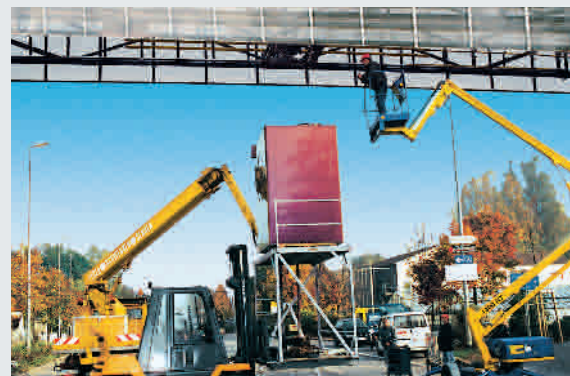
⑤ Installing the lift car
