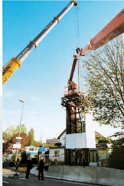
② Erection of the towers
